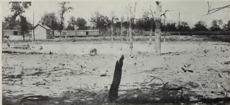
FIG. 28.—Pond 4 feet deep and covering an area of about an acre, due to subsidence near Clifford, where a coal bed about 7 feet, 6 inches is being mined at a depth of 140 feet. Considerable quicksand occurs in the vicinity. The rooms are driven 20 to 22 feet wide on 40-foot centers, and no pillars are drawn.
